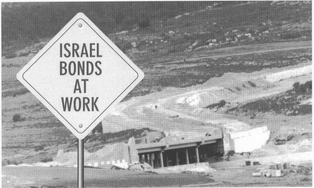
The Bet Shemesh Bridge, under construction in 1998, links the old city to the rapidly growing new city.
